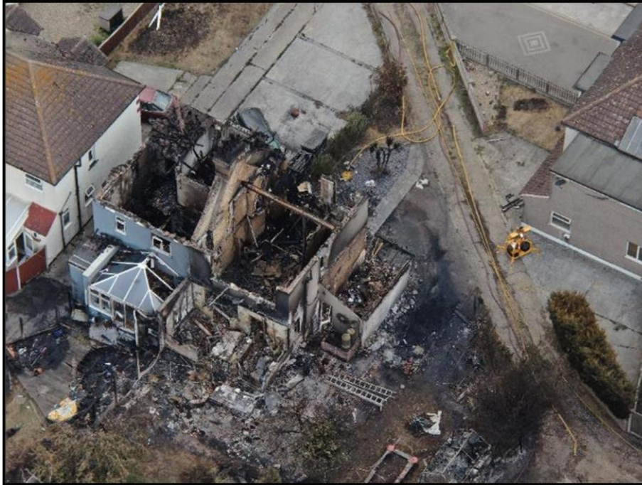
Image 3: No's.19 and 20 – viewed from the south
