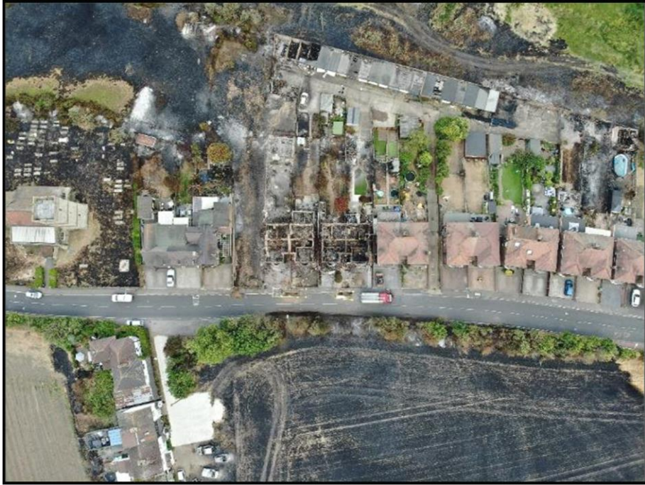
Image 7: Fire spread to Kent View
