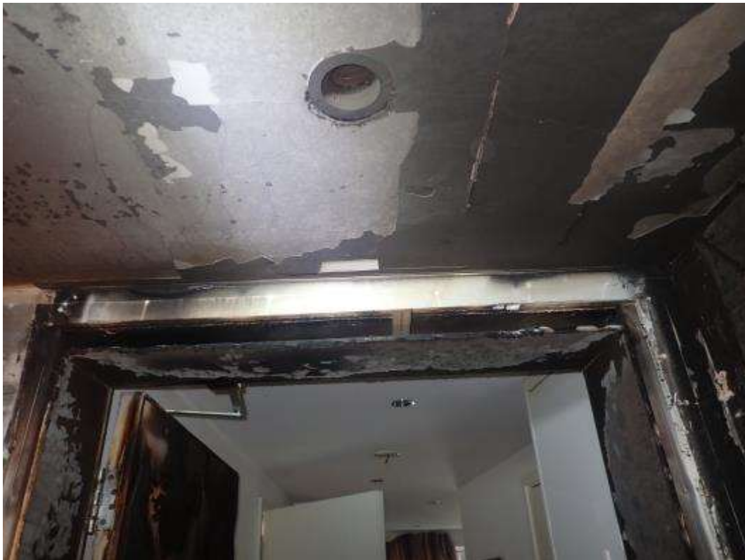
Image showing the void between the top of the door frame and the fabric of the building
