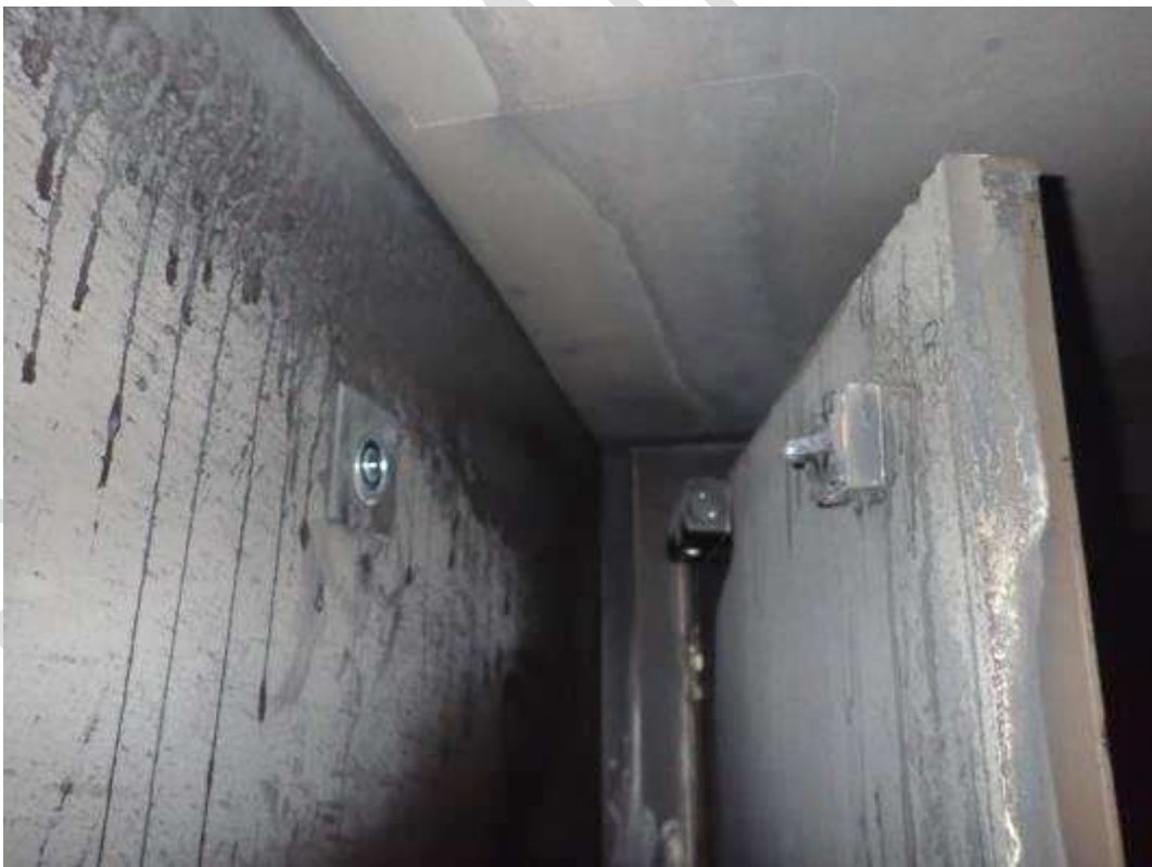
Image showing the magnetic holder for the cross corridor door on the 8 th floor
