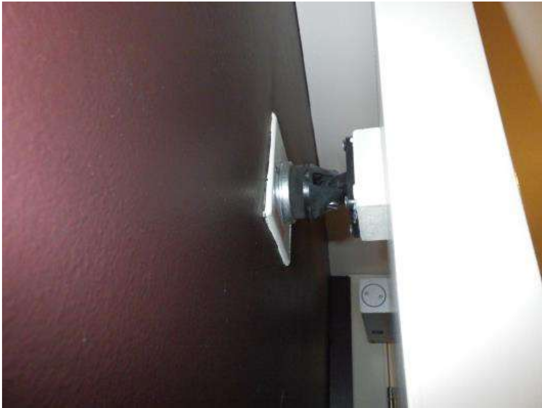
Image showing the magnetic holder for the cross corridor door on the 9 th floor
