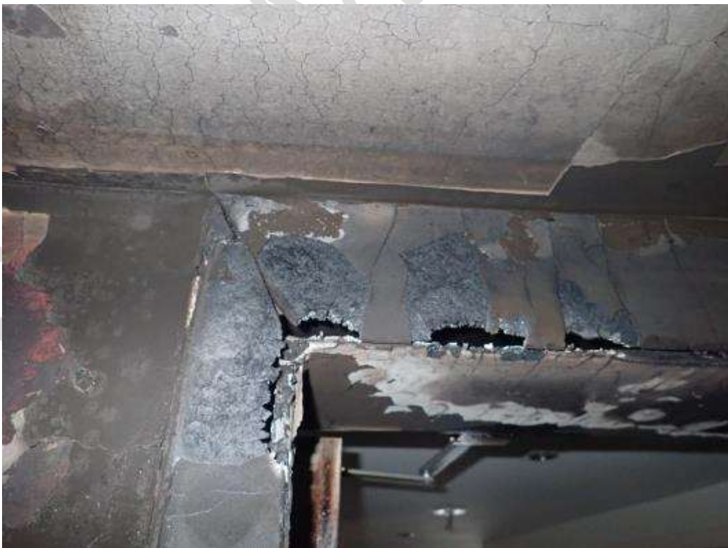
Image showing the timber boxing around the front door frame of flat next to flat of origin
