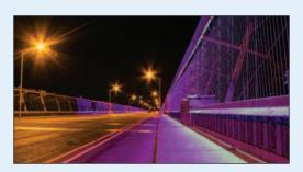
High-level suicide prevention barriers installed on the Prince Edward **Viaduct** in Toronto, Canada incorporated 450 metres of coloured LED lights, which change to reflect fluctuations in air temperature, as well as wind direction and velocity, creating a "living" piece of illuminated public art.
