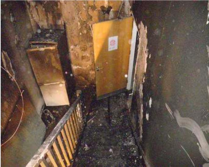
4.14 Fuelled by paper and stored goods, the fire started in the hallway on the ground floor offices at the base of the internal staircase to the flats (as shown in image to the left) and damaged approximately 50% of the ground floor. The remainder of the ground floor was damaged by heat and smoke, with the rest of the building damaged by smoke.
