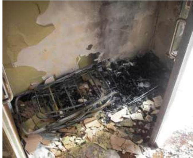
4.3 In another recent incident, a baby buggy was set alight on the ground floor of a common stairway area. Smoke spread up the stairway cutting off the single staircase escape from the upper floors.
