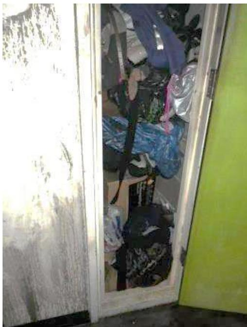
4.6 The three images on this page relate to a fire which occurred in a common lobby shared by 4 flats on the second floor of a high rise block. The seat of the fire was within a small cupboard (approximately 30-50cm wide) used to house services such as drainage and telephone cables. The cupboard had been filled with old clothes and electrical items (example image left).
