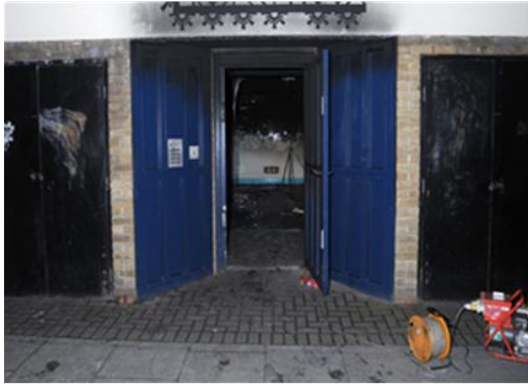
View of front communal entrance
